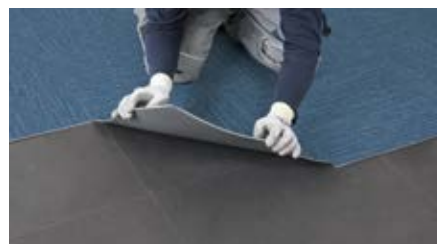
APPLY PLANKS OR TILES
